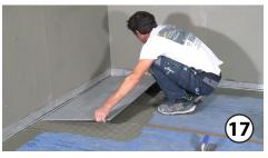
17. Apply **PRODESO SOUND TAPE** along the joints between rolls and install the floor on **PRODESO DRAIN 8**, with a trowel suitable for the tile size, by providing expansion joints in accordance with the rules.
